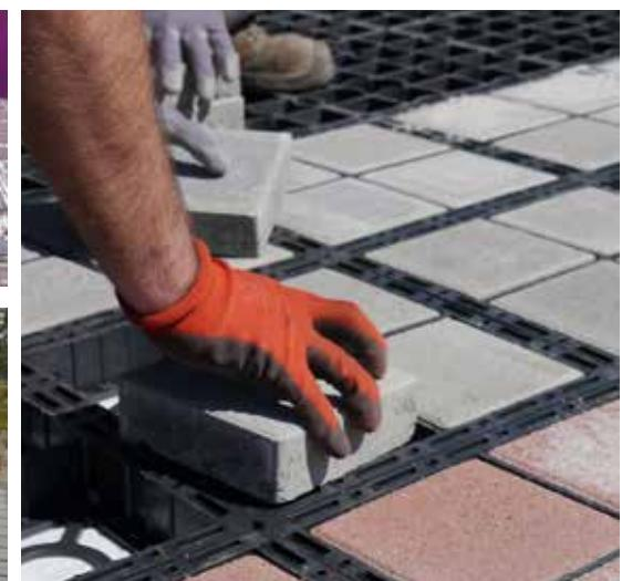
We recommend a subfloor structure and compression in accordance with the German road construction regulation RStO.
